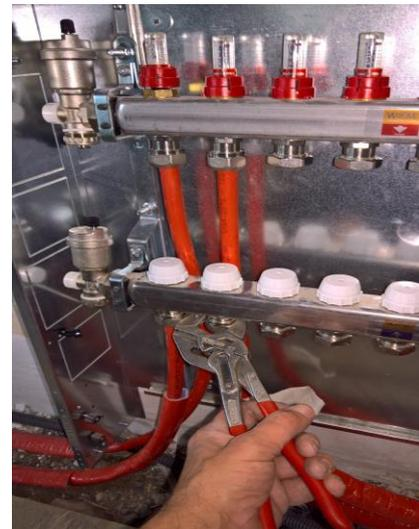
Seal unused manifold connections with safety caps.
