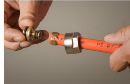
Push the fitting body into the pipe until it stops.
